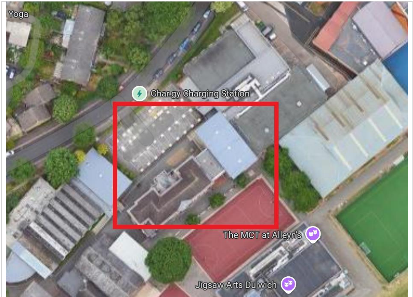
Aerial View of Building
