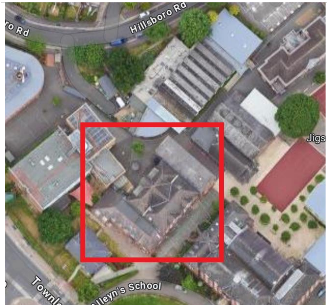
Aerial View of Building
