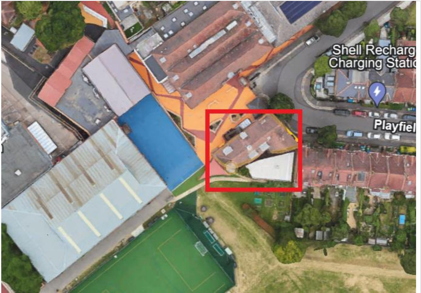
Aerial View of Building
