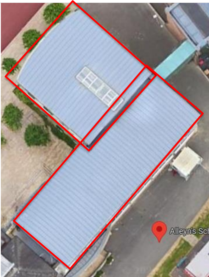
Aerial View of Building
