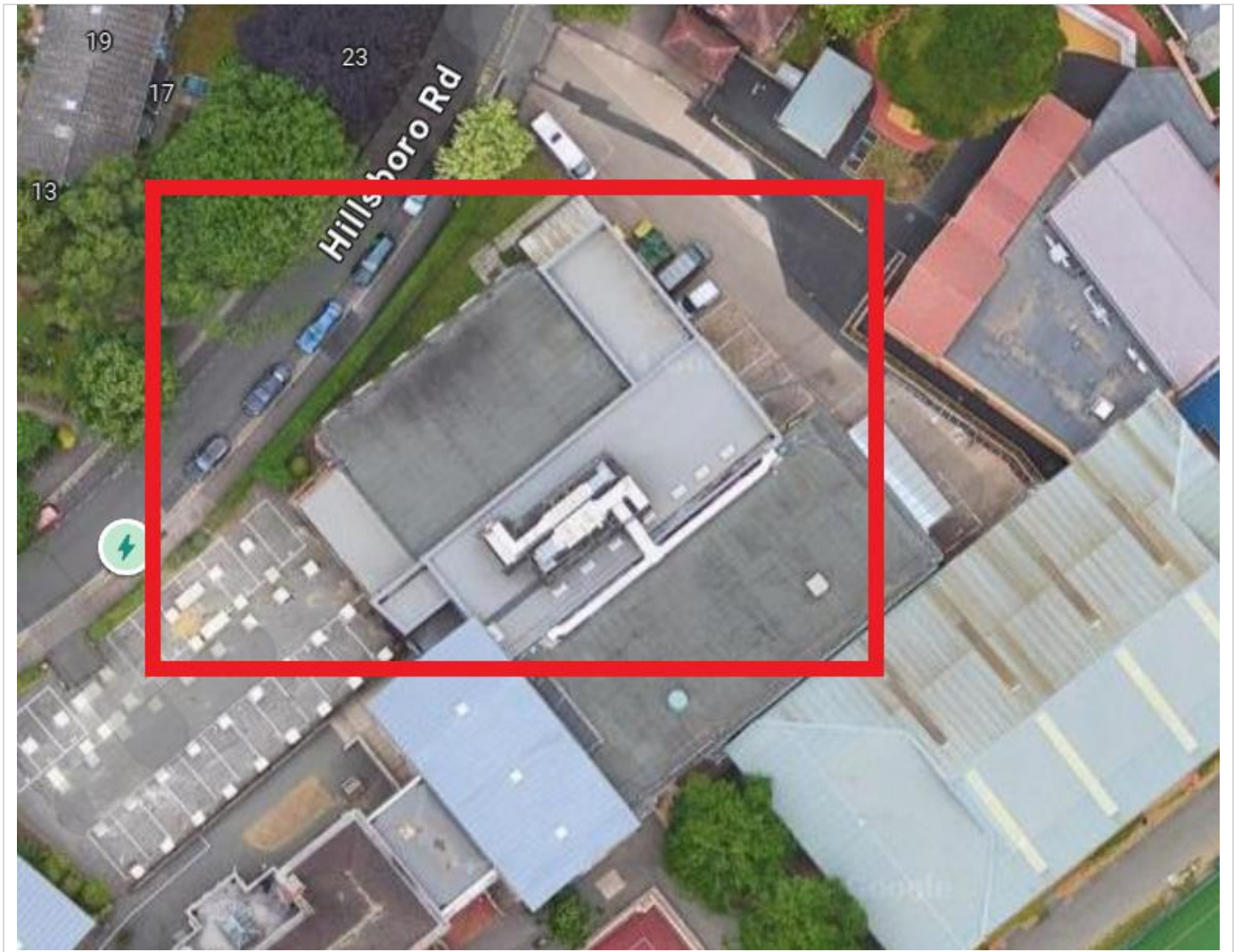
Aerial View of Building
