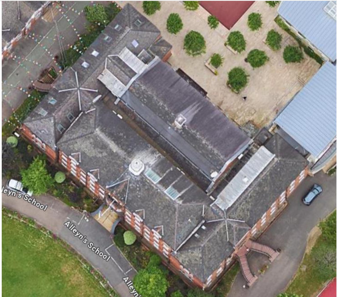
Aerial View of Building
