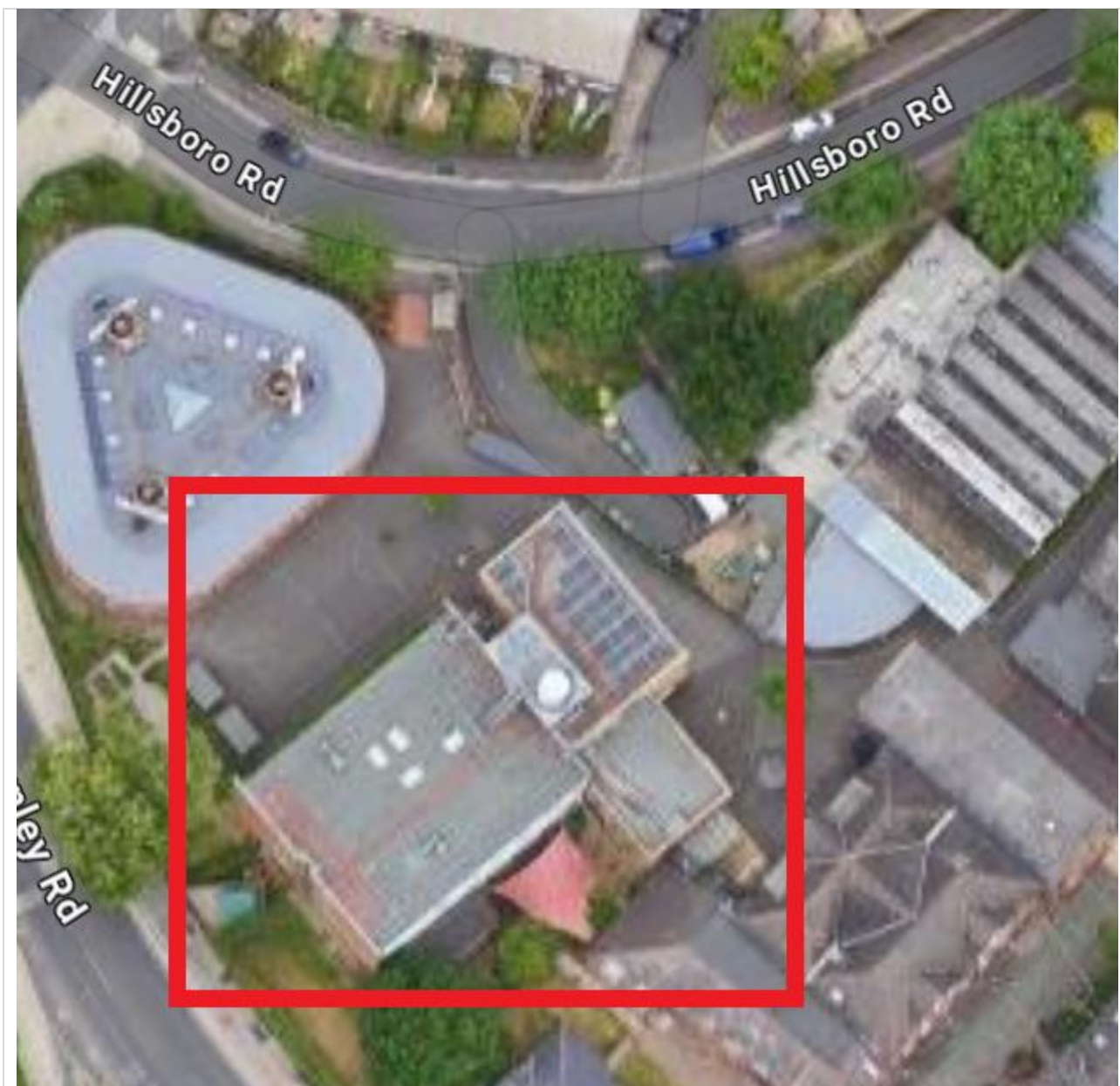
Aerial View of Building
