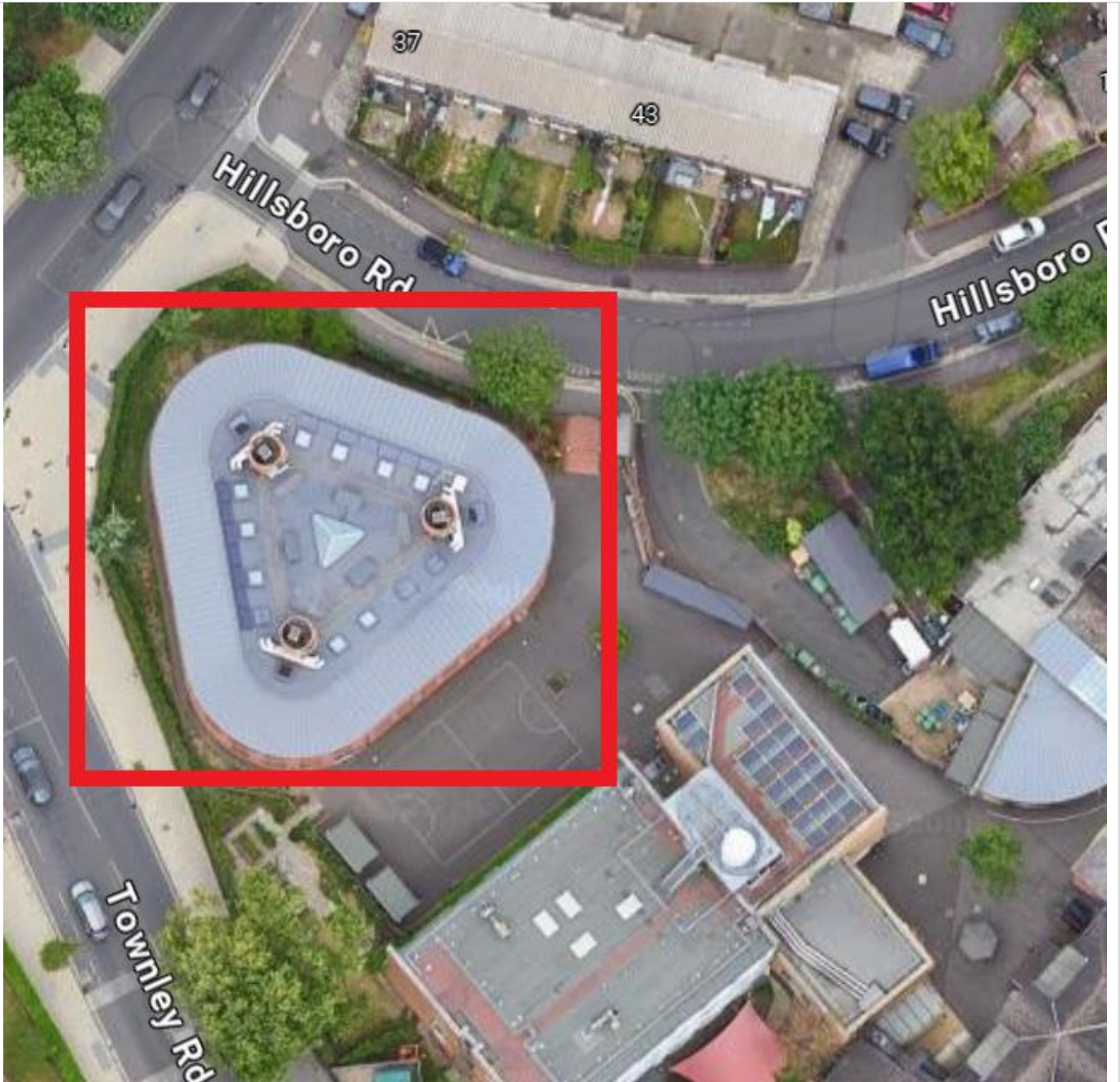
Aerial View of Building
