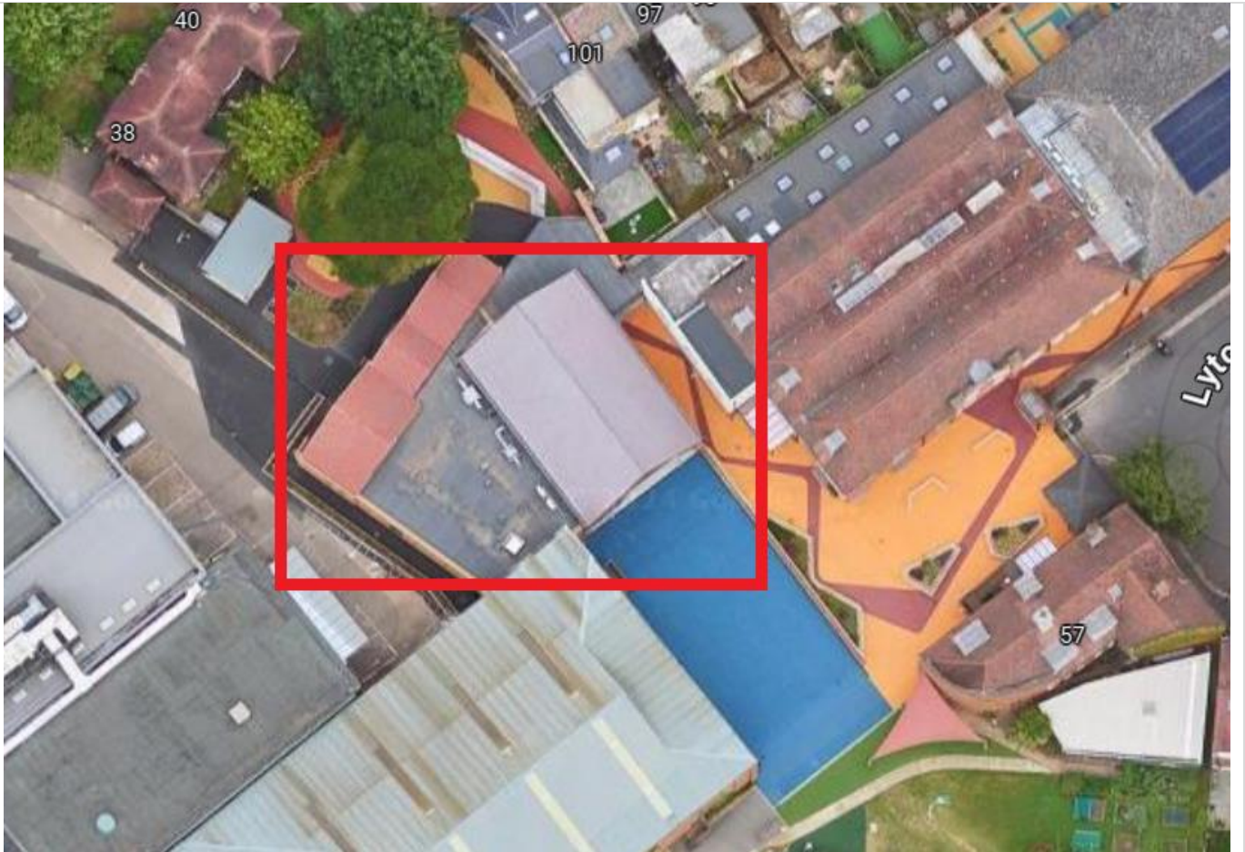
Aerial View of Building
