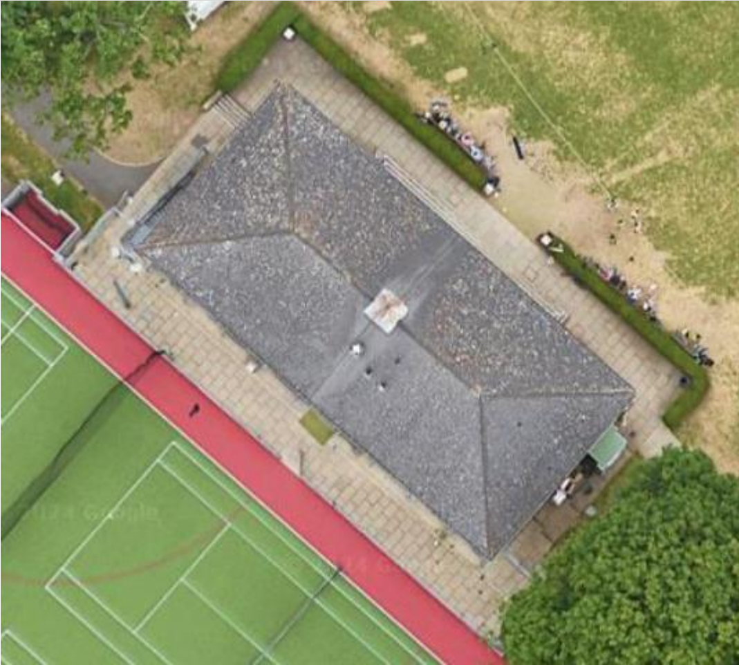
Aerial View of Building
